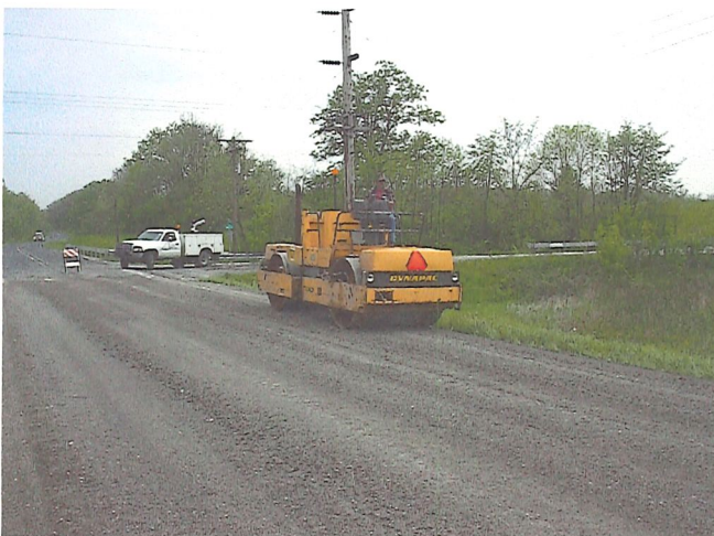
Compacting Surface
