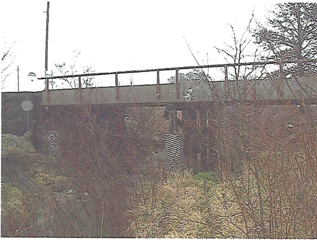
Old Bridge (Closed)
