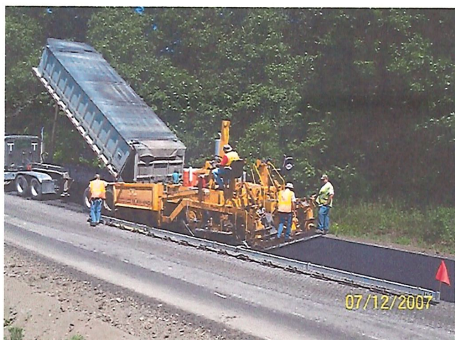
Resurfacing Pavement
