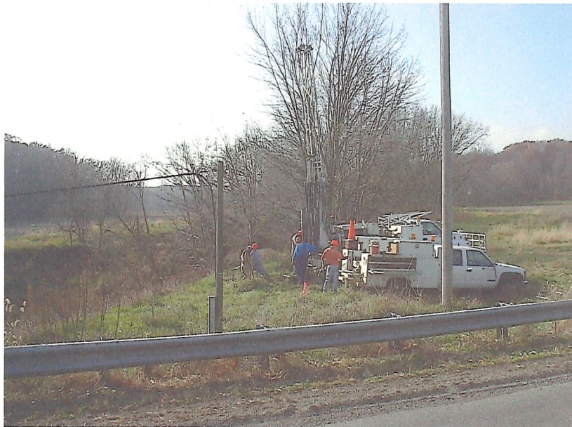
Soil Boring at Major Bridge (near Mode) along County Highway
