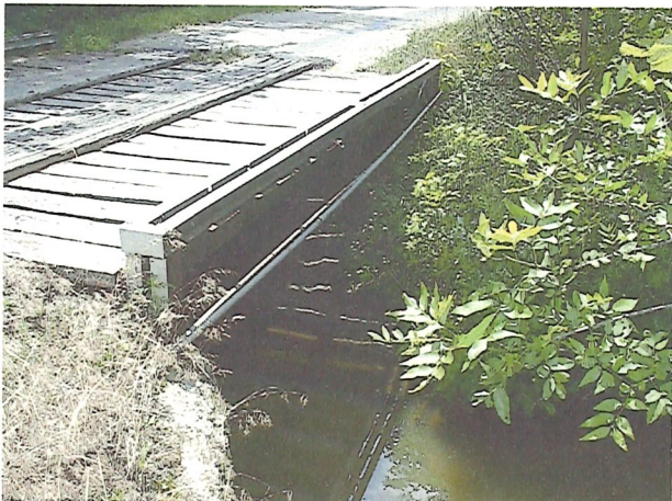
Old 3 ton Posted Structure
