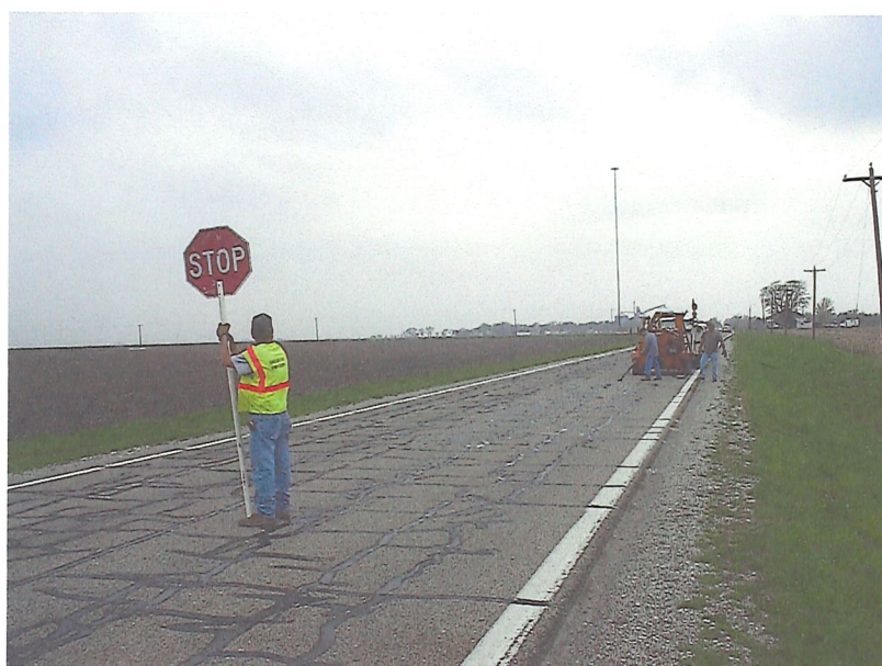
Crack Sealing the Bruce-Findlay County Highway
