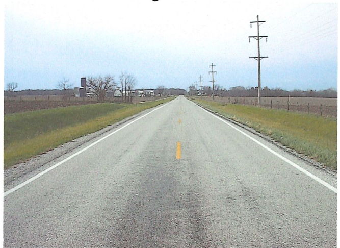
Final Road Surface
