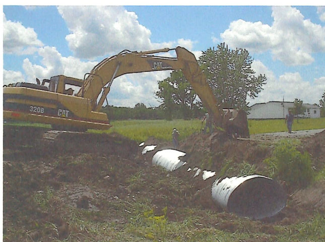
Lakewood County Highway Pipe Replacement
