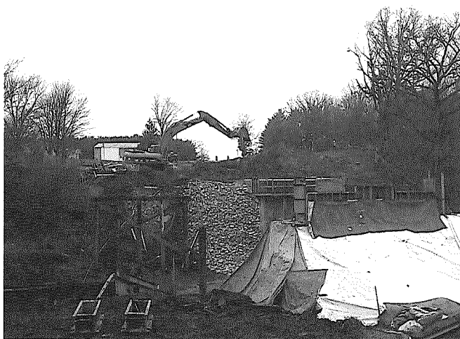
Bridge Under Construction
