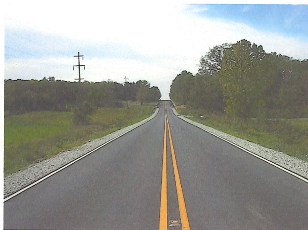
Final Road Surface
