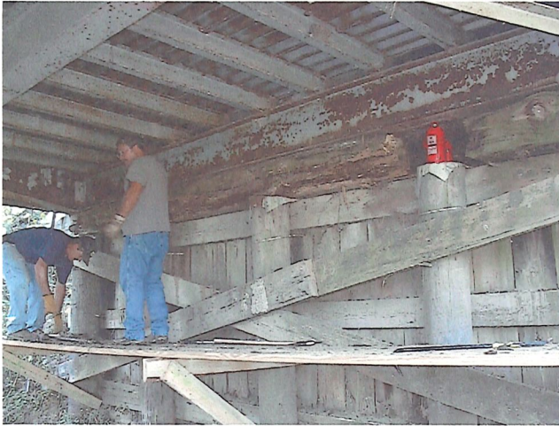
Repair of Deteriorated Cap
