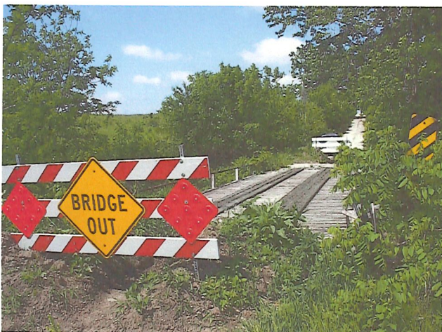
Old Bridge (Closed)
