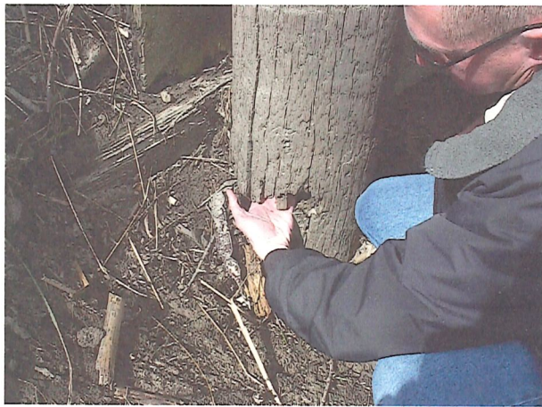
Bridge Inspection (Closed Bridge)
