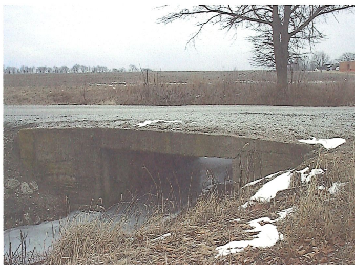
Existing Box Culvert
