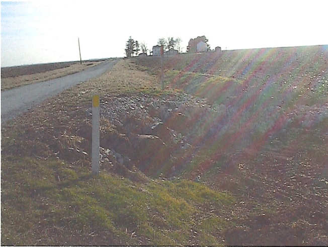
Old Pipe Culverts
