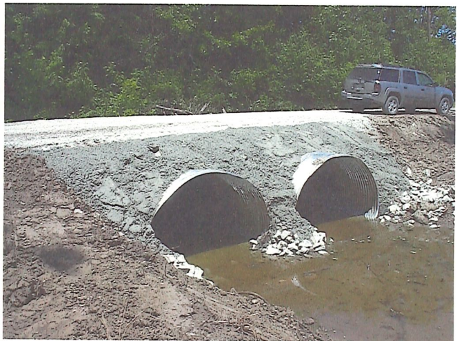
New Pipe Culverts
