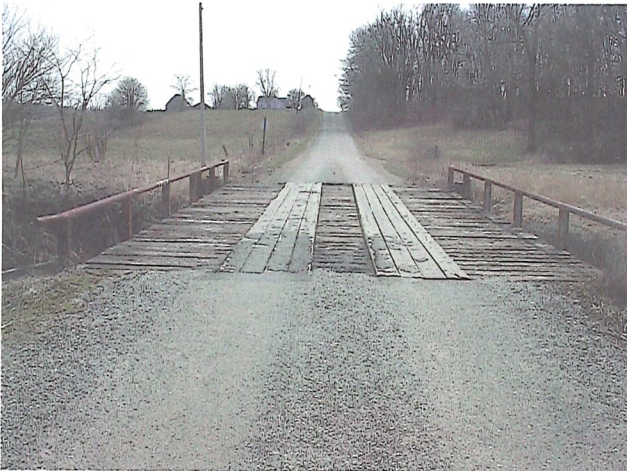
Old 5 Ton Posted Bridge
