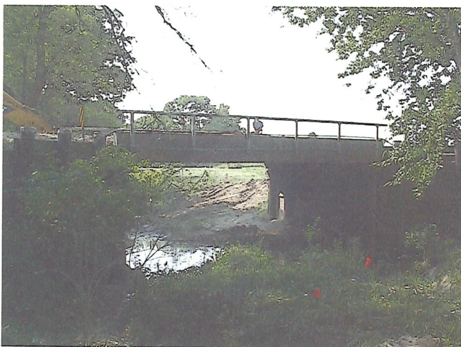
Old 5 Ton Posted Bridge
