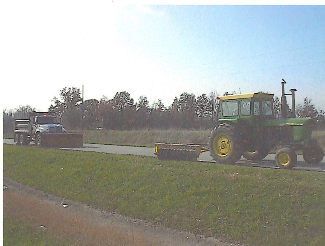
Repairing Shoulders along Cowden-Herrick County Highway
