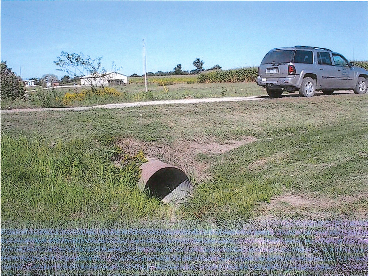
Ridge Township 1250E-1550N need 42 inch by 40 feet
