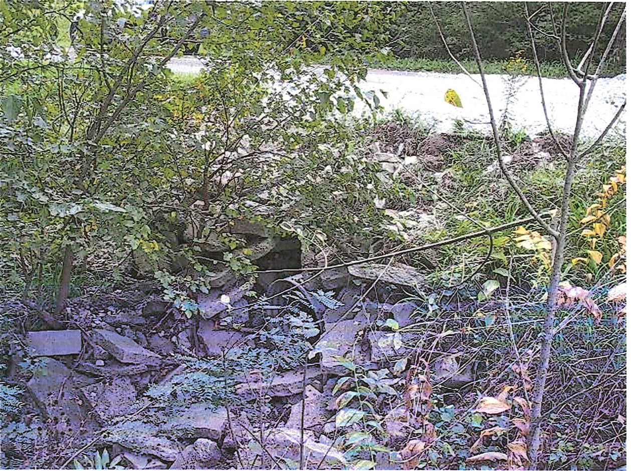
Lakewood 50-50 550n - 1650e 36 inch x 38 feet
