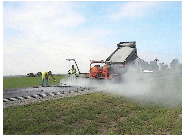
Patching Repairs for Moweaqua County Highway
