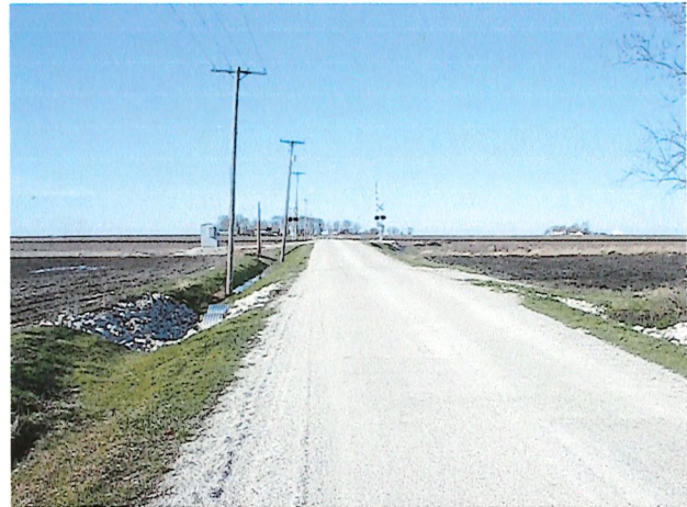
Finished Approach at 1650N
