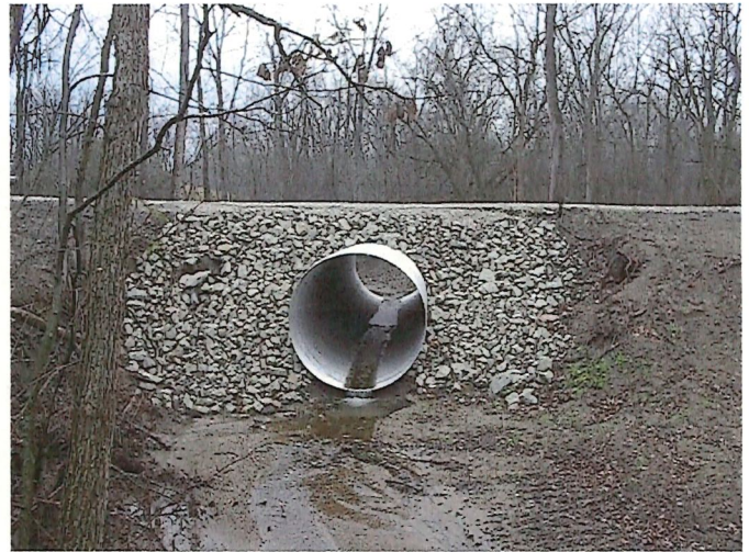
New Pipe Culvert
