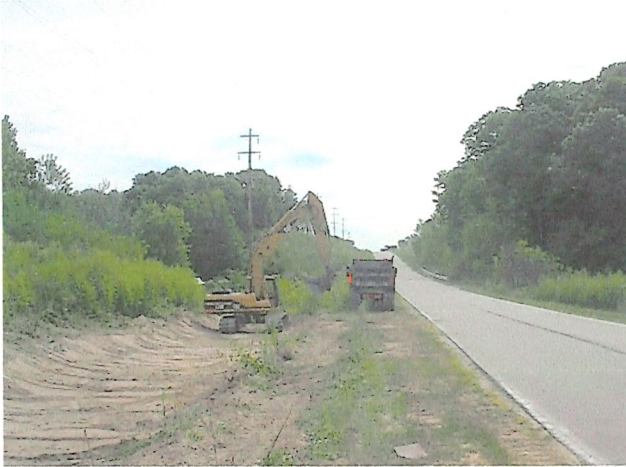
Ditch Cleaning along Oconee-Nokomis Road
