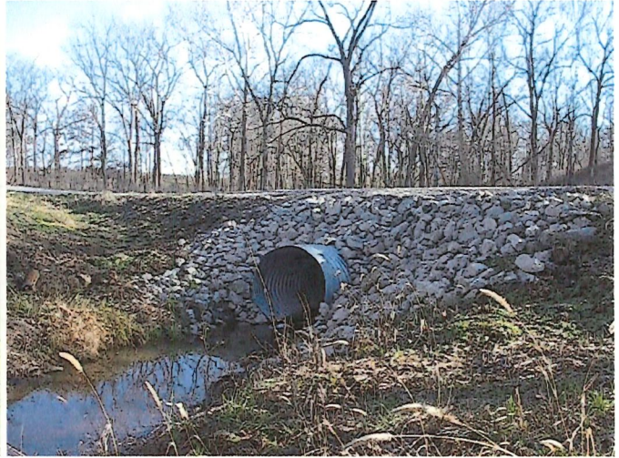
New Pipe Culvert
