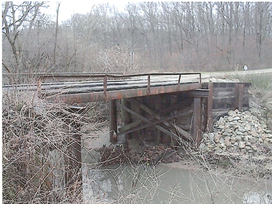
New Steel Beam and Steel Piles
