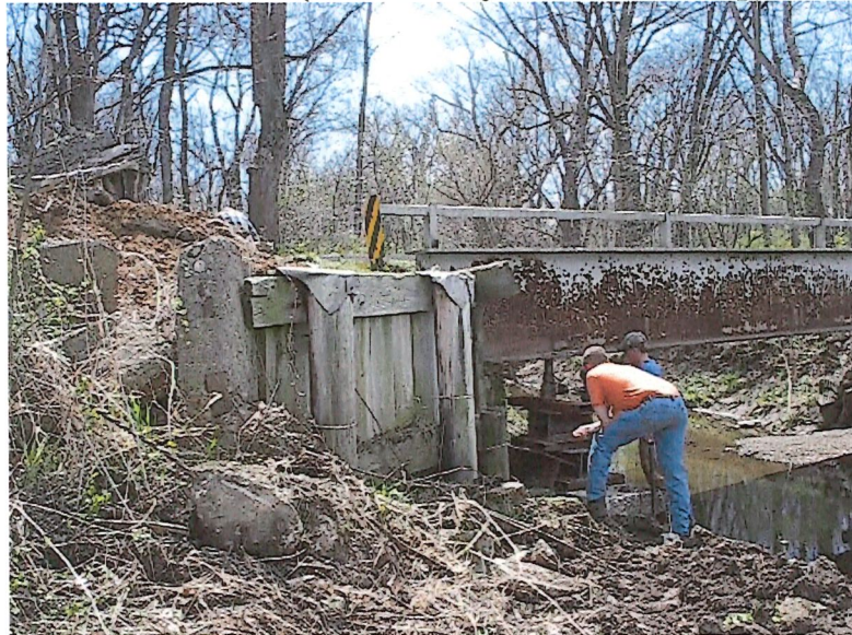
New Pier Caps
