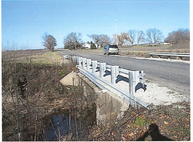
Repaired Bridge Rail
