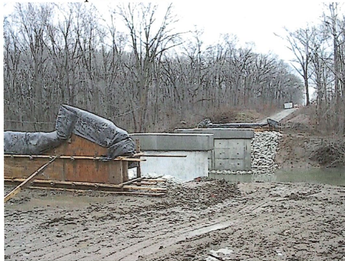
Bridge Construction in Progress
