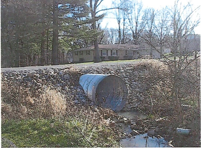
New Pipe Culvert
