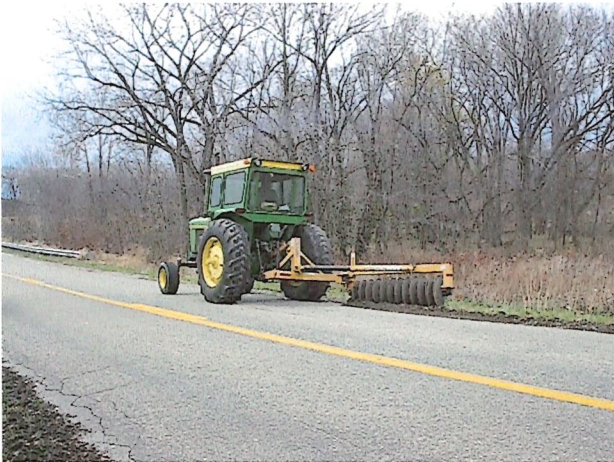
Shoulder Repair for Clarksburg Cty Highway
