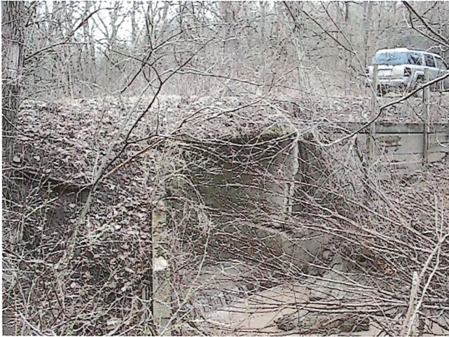
Existing Box Culvert
