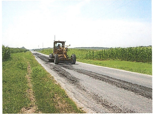
Cold Mix Overlay for Vandalia County Highway
