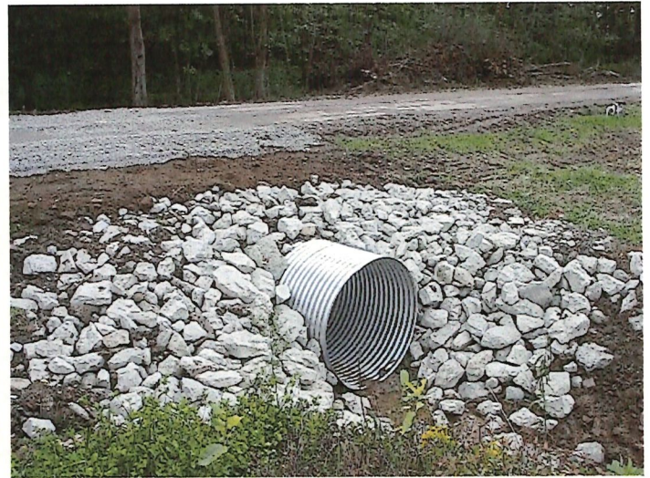
New Pipe Culvert
