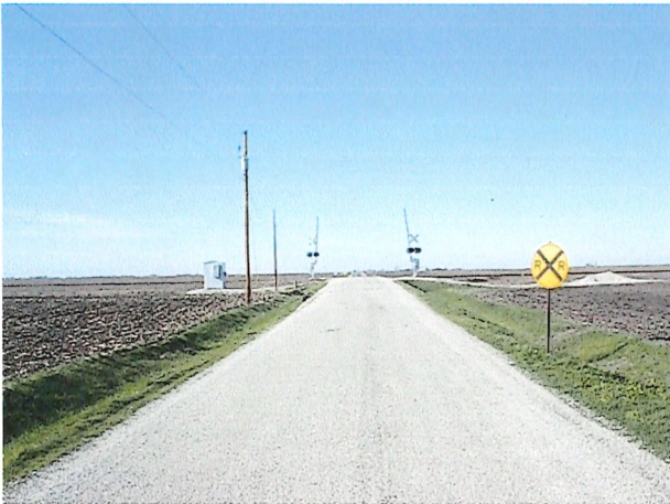
Finished Approach at 1600N
