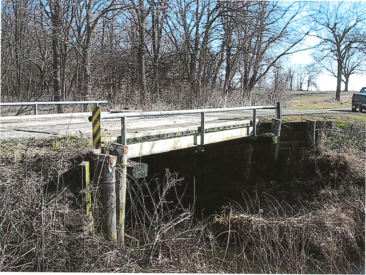
bridge existing 087-3351 richland (640x480x24b jpeg)
