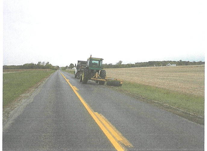
Shoulder Repair: Tower Hill-Moweaqua Cty Hwy
