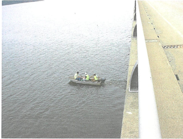
Underwater Inspection of Findlay Bridge crossing Lake Shelbyville
