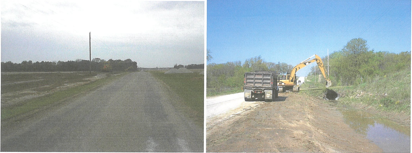
Ditch Cleaning along Oklahoma and Neoga County Highways
