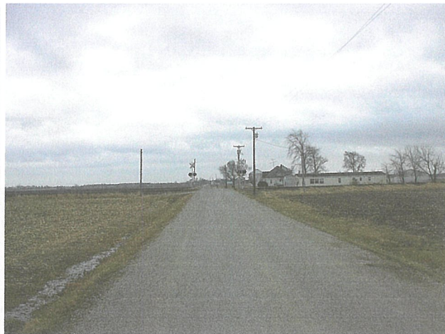
New Road Approach
