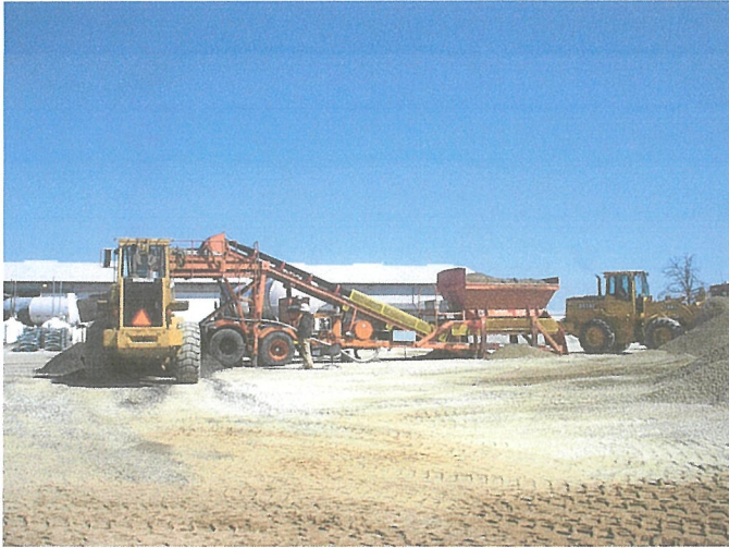
Make Cold Mix for County and Townships
