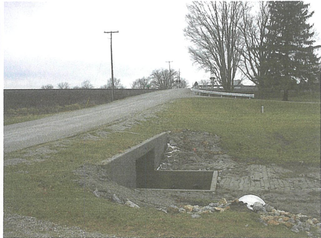
New Road and Box Culvert
