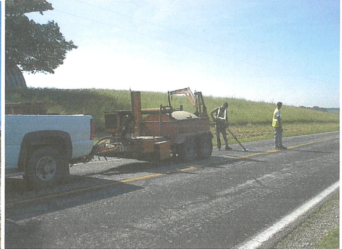
Crack Sealing of Tower Hill-Herrick Cty Hwy
