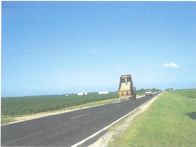
Repair Edges of Mowequa County Highway
