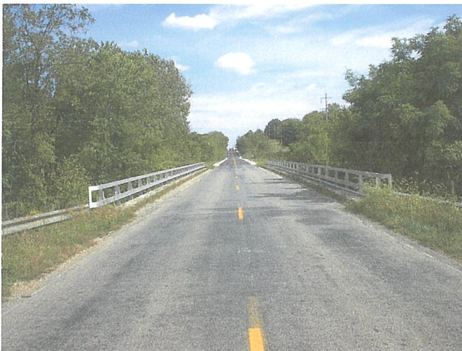
Existing Bridge (33 Ton Posting)
