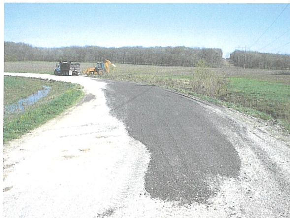
Repair Herrick-51 County Highway due to Flood Damage (FEMA funded)
