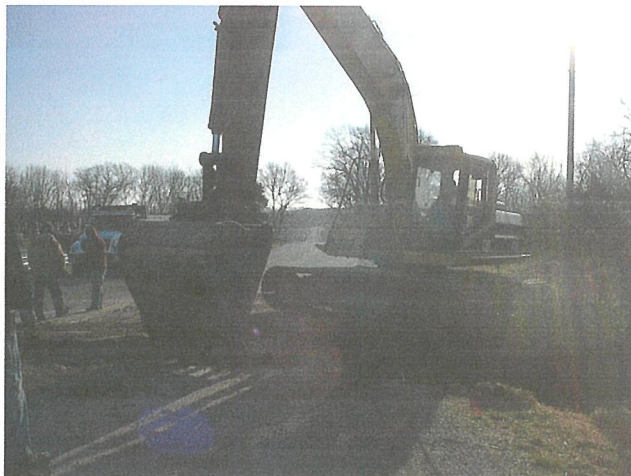
Replace Pipe Culvert across Clarksburg Blacktop
