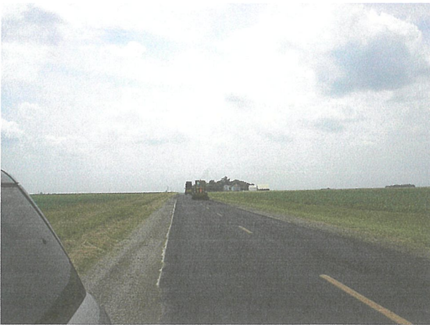
Leveling/overlay of Moweaqua Cty Highway
