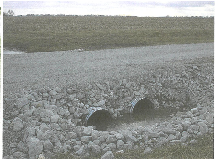
New Pipe Culvert
