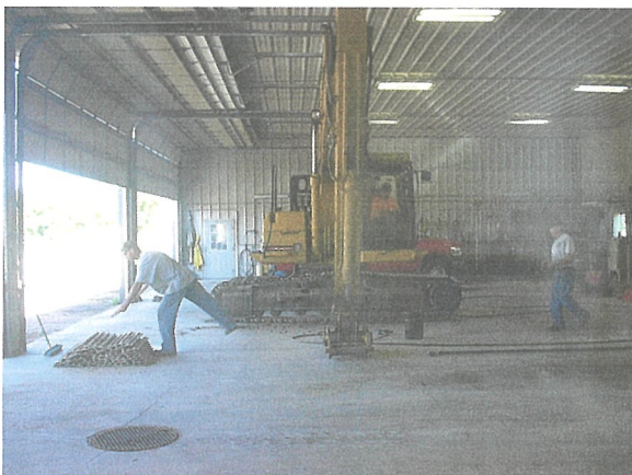
Replace Tracks on Excavator
