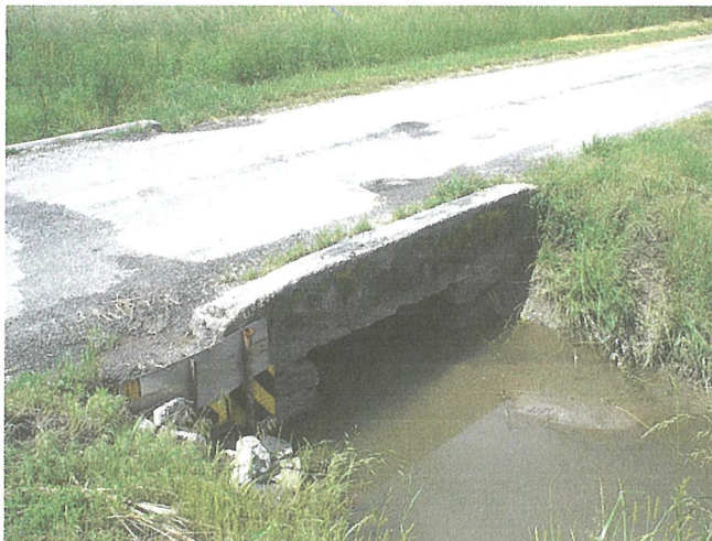
Existing Box Culvert
