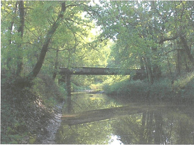
Old Bridge (Closed)
