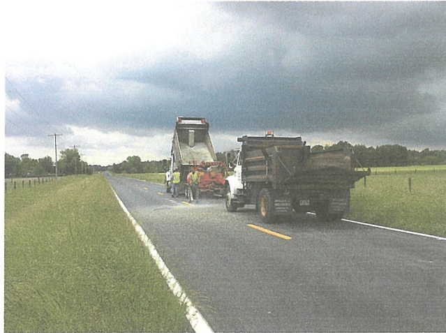
Patching Repair along Coon Creek County Highway
