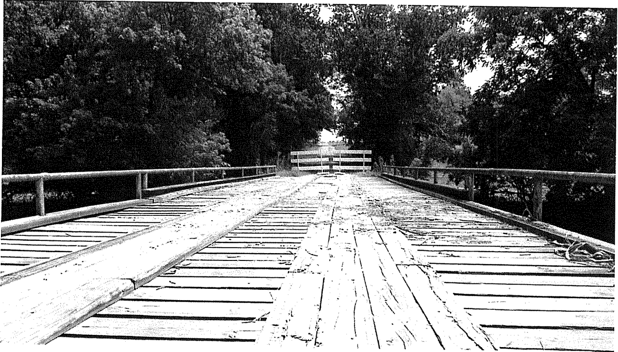
Standing at West Abutment, facing East. Debris has been removed from under deck boards.
