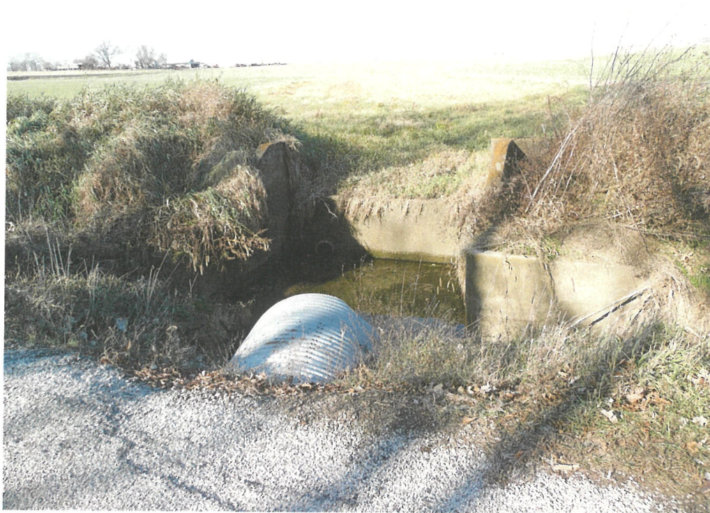
Ash Grove 1300N 3100E Existing pipe is 60" x 36 feet
