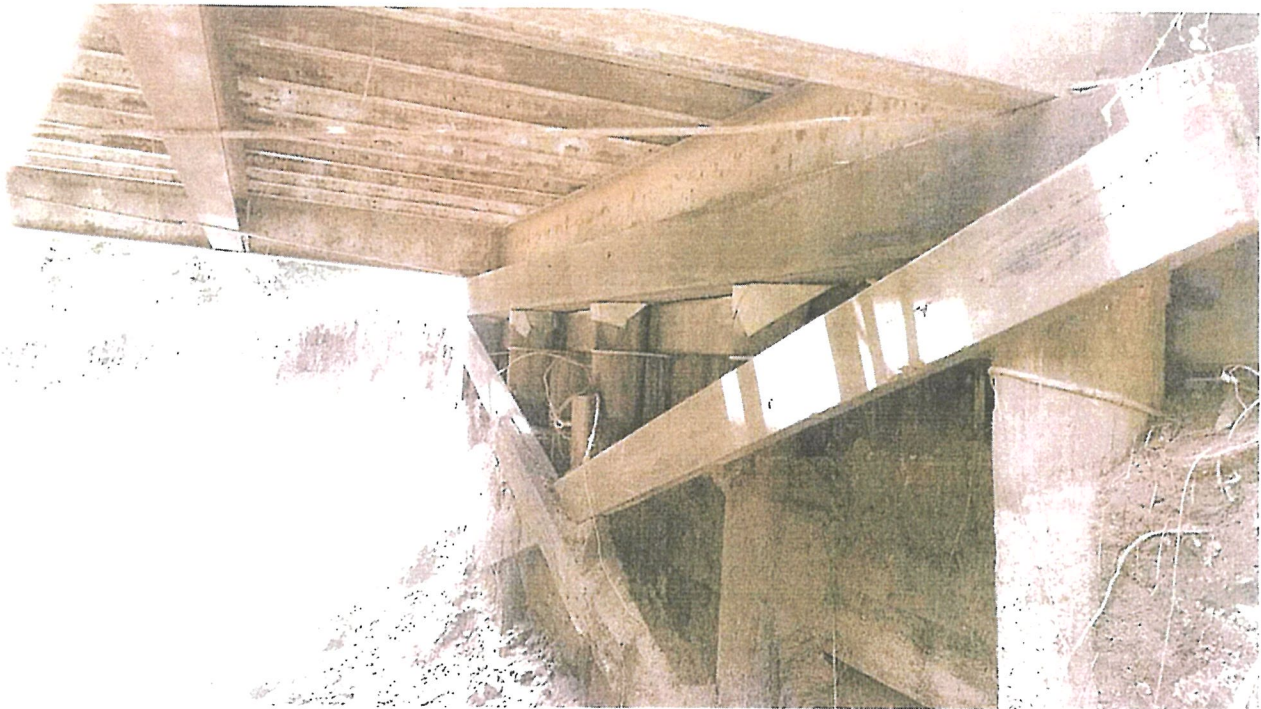
West Abutment, facing South.
