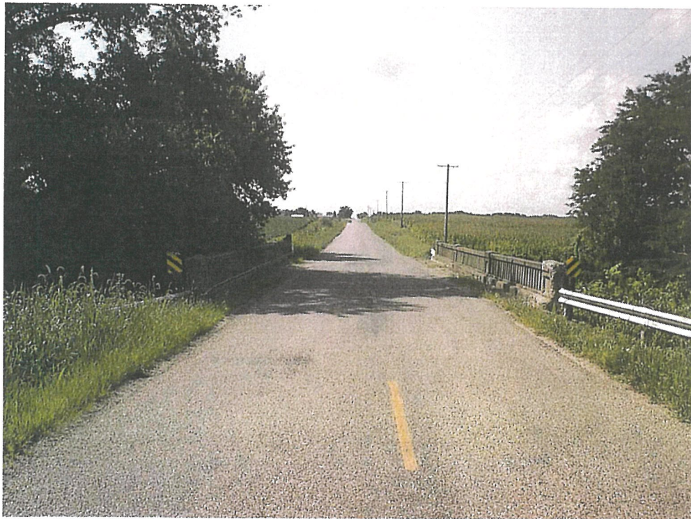
Westervelt County Highway #41 087-3016 - Major Bridge Program
