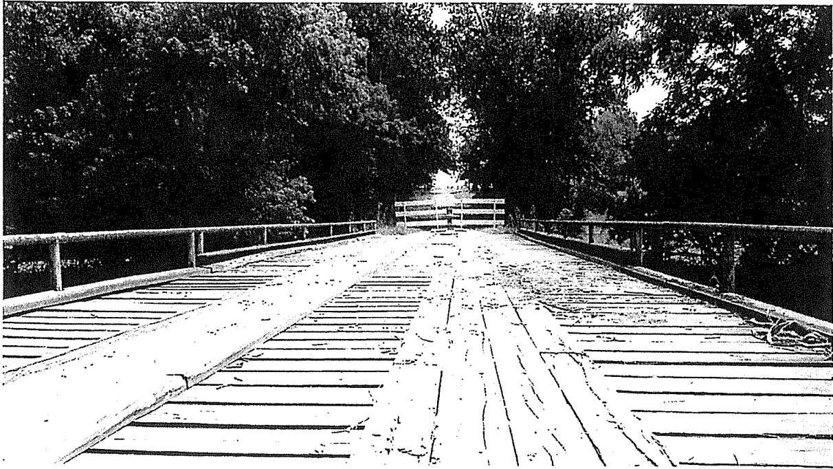
Standing at West Abutment, facing East. Debris has been removed from under deck boards.
