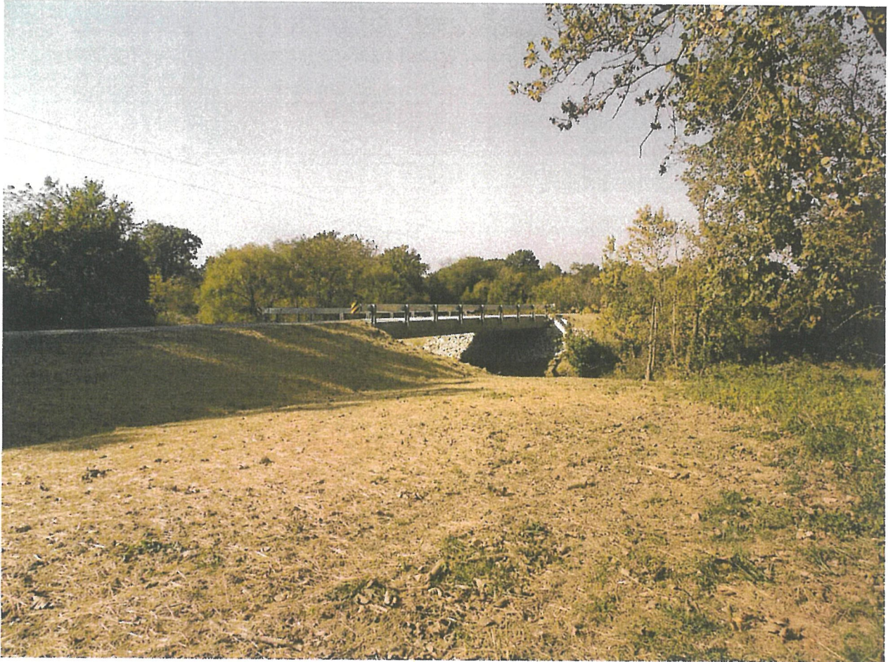
Prairie Bridge Completed 087-3593
