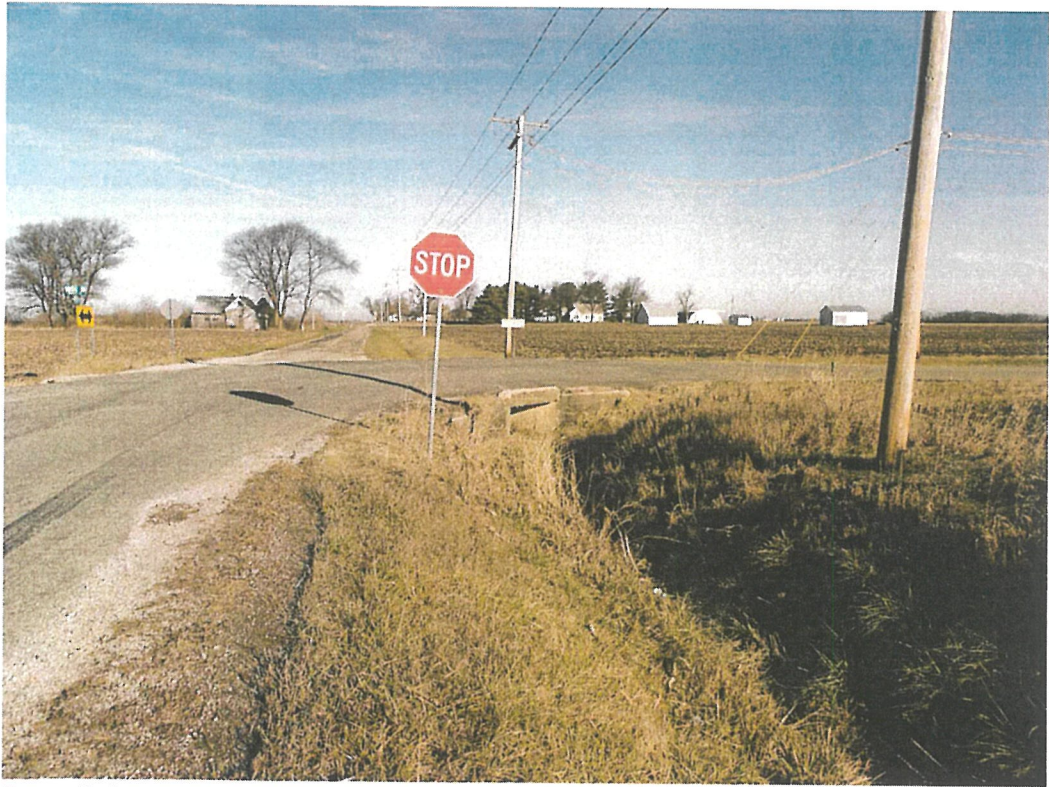
Duvall Corner on Country Club Road – CH #5
