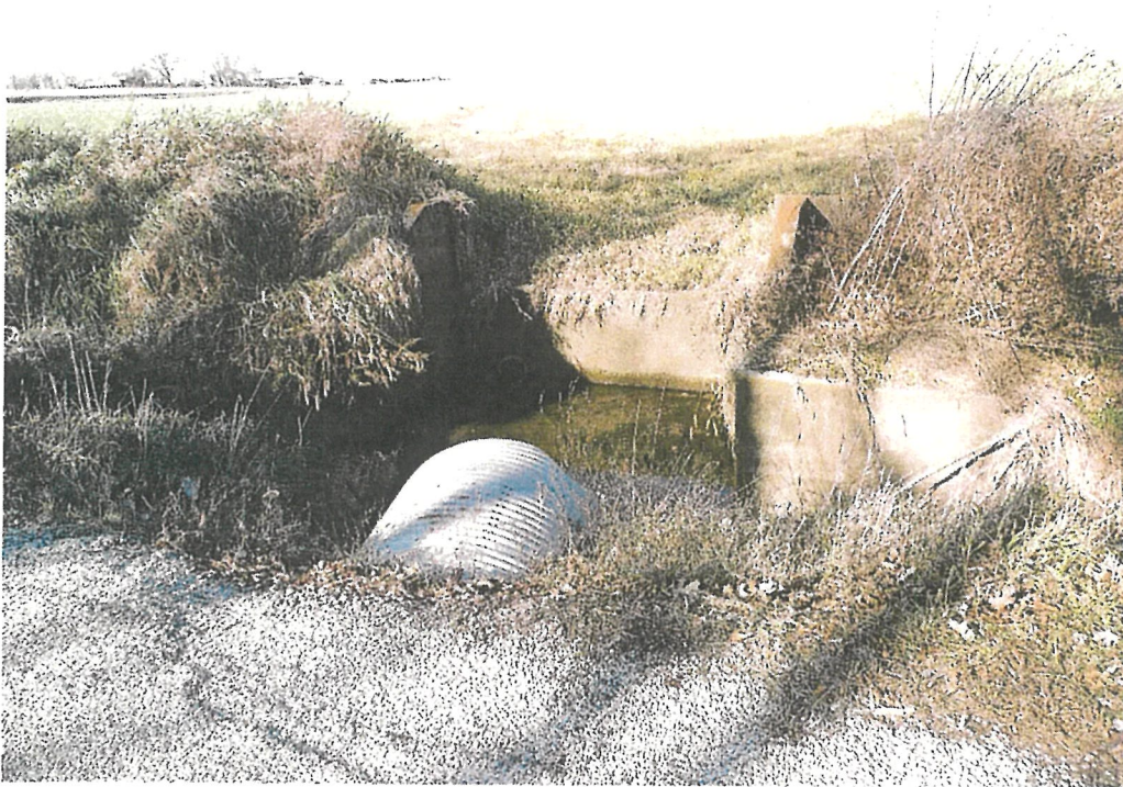
Ash Grove 1300N 3100E Existing pipe is 60" x 36 feet
