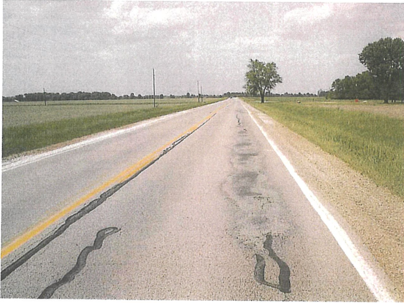
Cowden-Herrick Road Resurfacing Project
