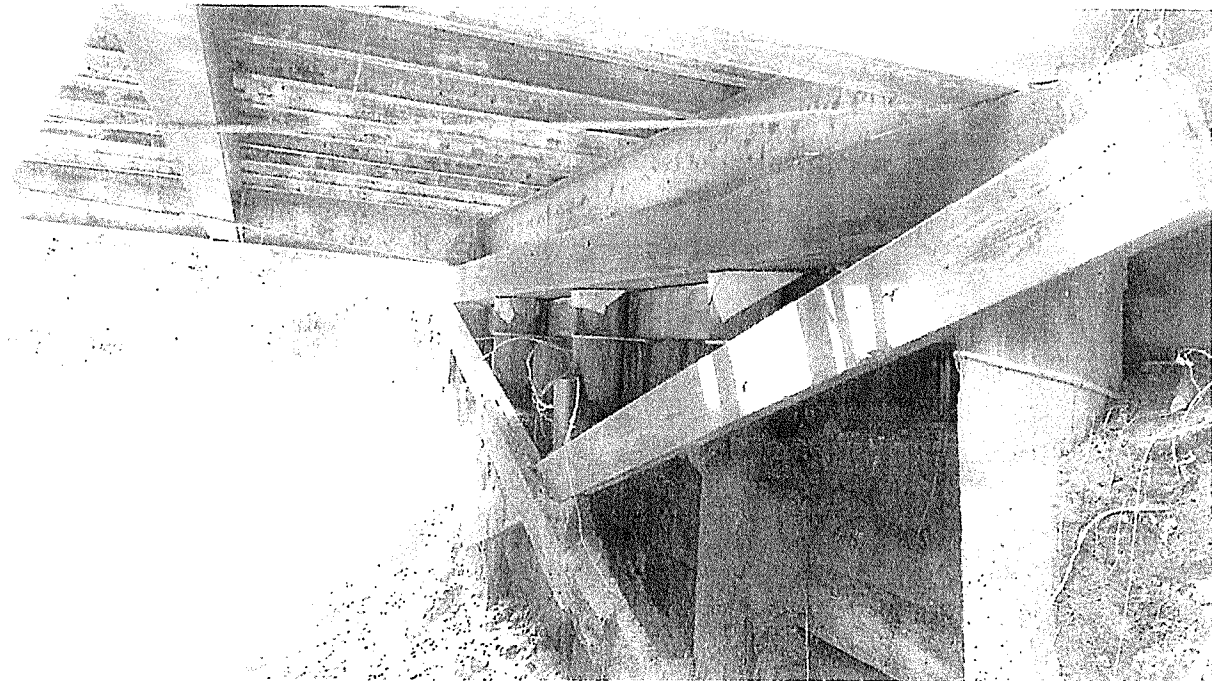
West Abutment, facing South.
