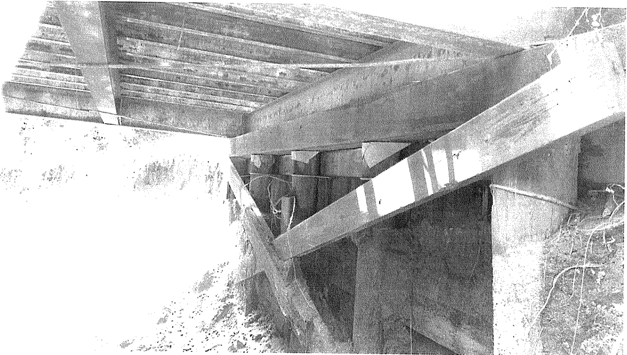
West Abutment, facing South.
