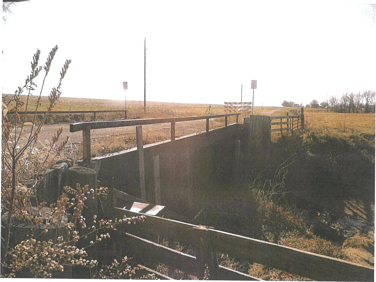
Flat Branch Bridge – 087-3101 - Closed 2525N 1100E
