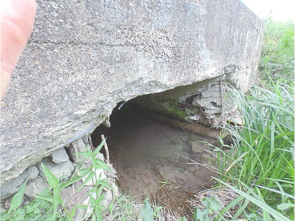
View on upstream side, facing southwest
