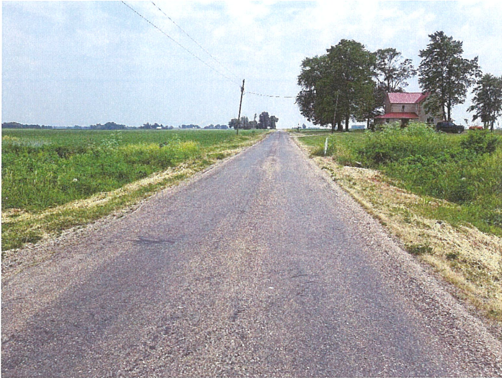
View along centerline, facing south
