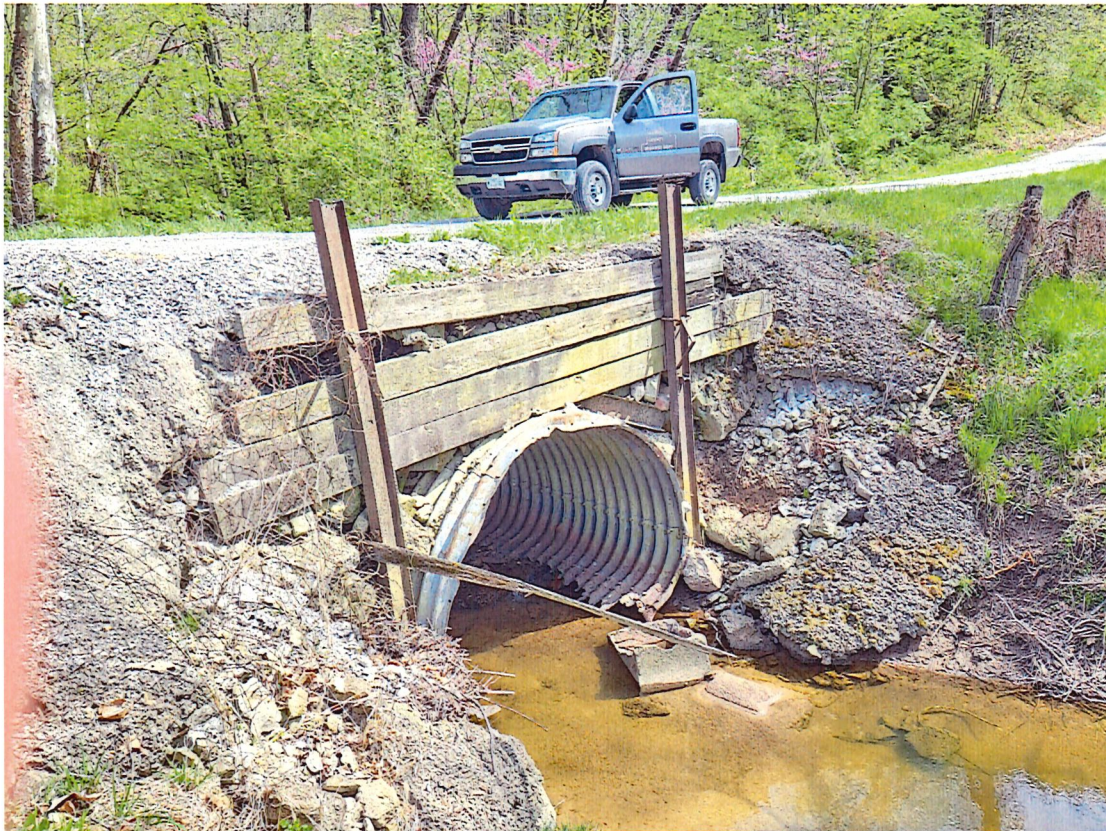
Downstream End, facing East
