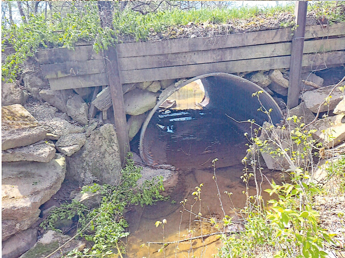
upstream end, facing west
